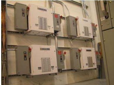
Solectria Renewables inverters up and running.
